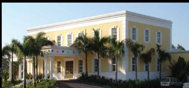
Bahamas Headquarters & International Sales Office
